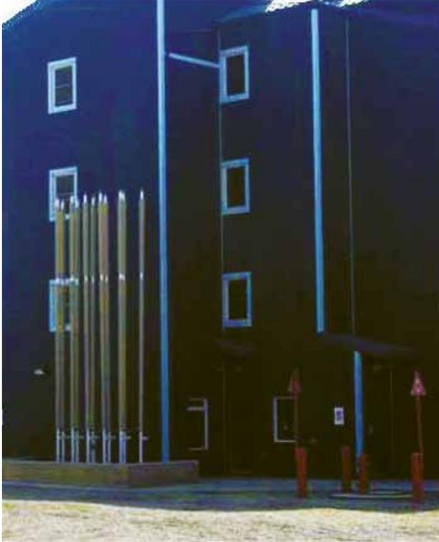
**Appendix F10.** *Thermosyphons are an example of a foundation system that requires significant expertise to design, install, maintain, and monitor (Barriault, 2012).*
