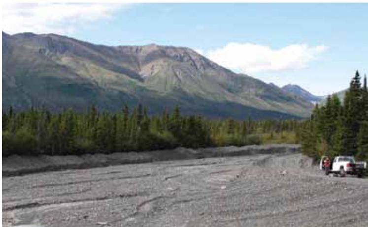
**Figure 28.** An example of berms on Bock’s Creek that serve to mitigate potential debris floods and flows.
