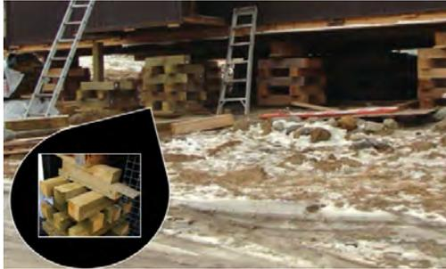
Maintenance operations are almost the same as for screw-jack foundations, described above; however, the operator must use a hydraulic jack to lift the load of the building before shimming the timber blocks. Maintenance for this style of foundation is therefore more labour intensive than for screw-jack foundations.
